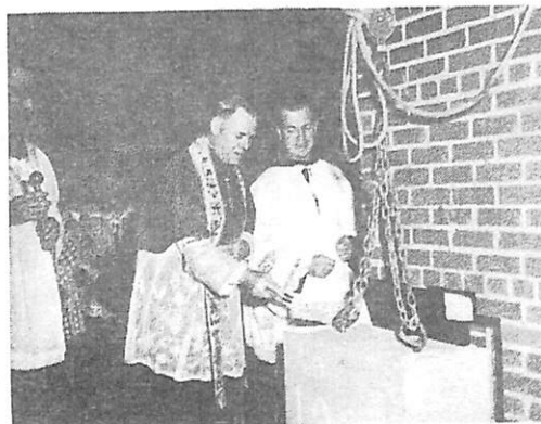
Laying of the cornerstone by the Most Reverend Francis J. Haas, Bishop of Grand Rapids at the Sisters Convent February 17, 1952.
