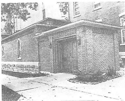
In 1978 a ramp was built to accomodate the handicapped. In the corner of the photo is part of the Friary.
